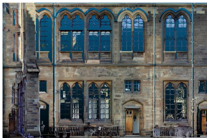
Img. 05.05. Visualisation of Point clouds with iSTAR data using Leica cyclone to colourisation in 3rd party software.
