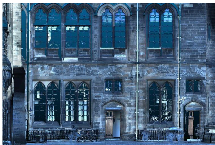
Img. 05.06. Visualisation of Point clouds with laser scanner internal camera data using Leica cyclone to colourisation in 3rd part software.
