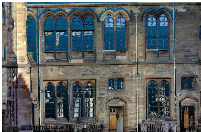
Img. 05.04. Visualisation of Point clouds with iSTAR data using NCTech ColourCloud in 3rd party software.
